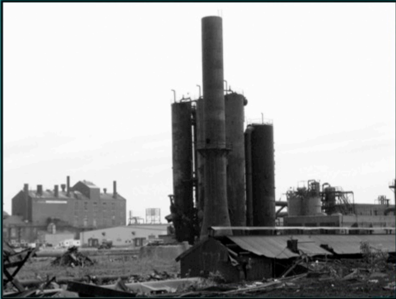
Bethlehem Steel Warehouse
