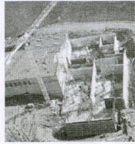
New Reservoirs under construction
