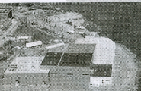
Plant nearing completion
