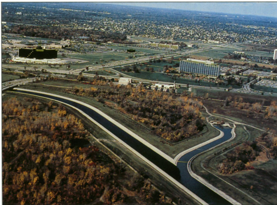
A portion of the concrete channel (constructed for flood control) in the main branch of the Rouge River, Dearborn, Michigan. Note the Detroit-Dearborn Channel which enters the main branch. Annual combined sewer overflow volume entering this channel is approximately 22 million m 3 . Photograph courtesy of Southeast Michigan Council of Governments.
