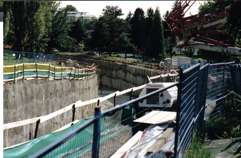
SkyTrain Extension ( Canada Line to airport) Under Construction June 2006
