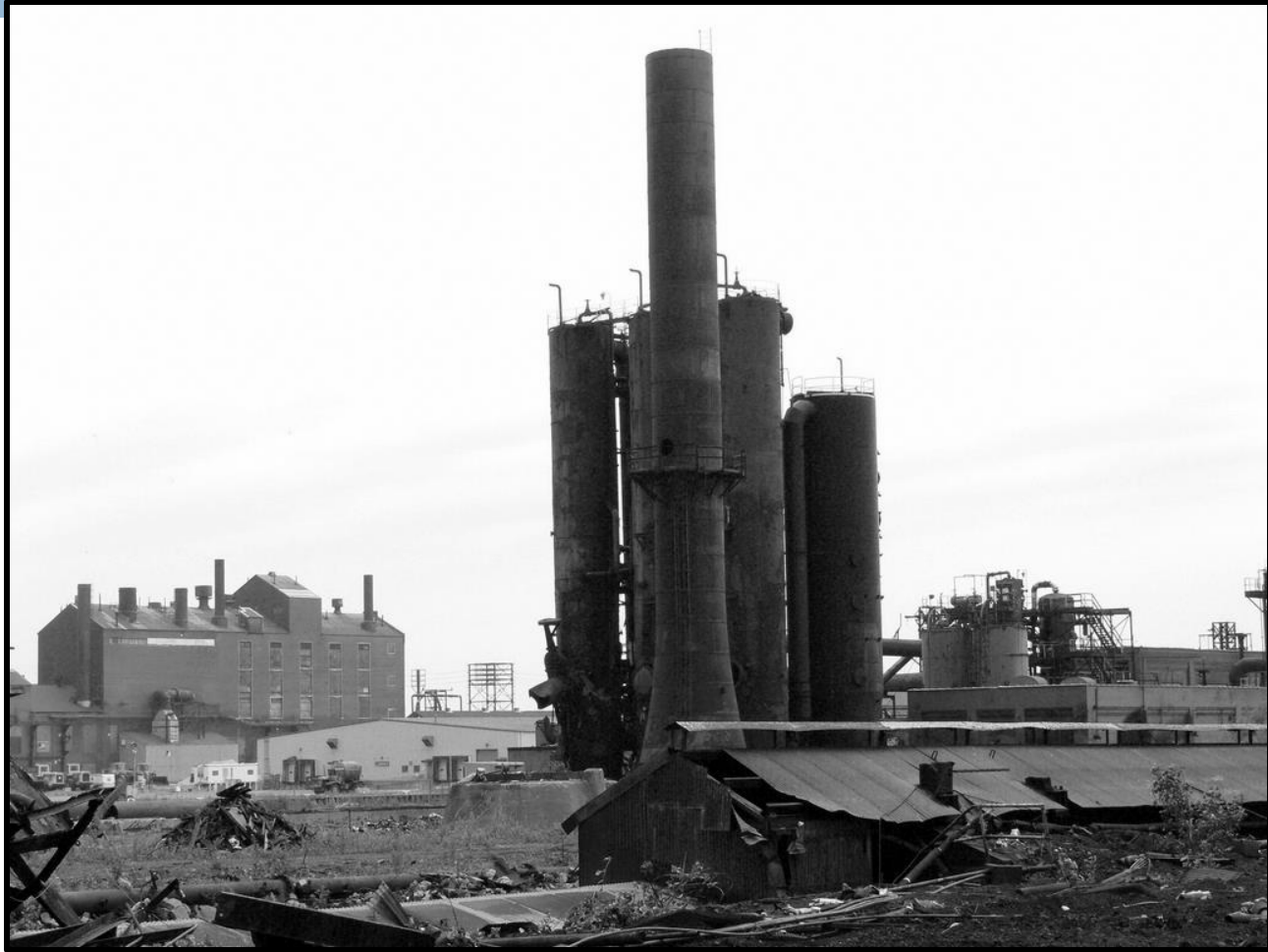
Bethlehem Steel Warehouse
