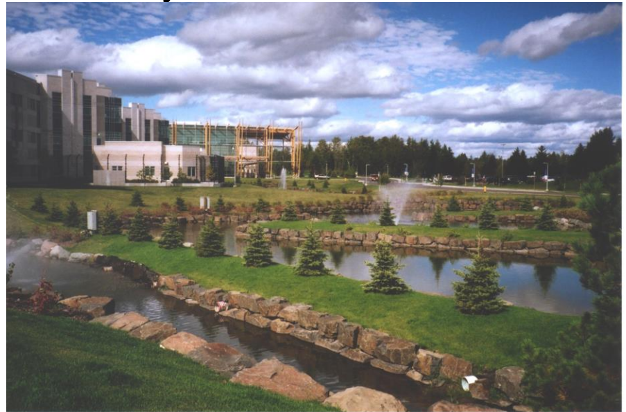
Series of retention ponds along east side of TBRH structure. Fountains to reduce/prevent mosquito larvae. TBRH site (Fall 2004).
