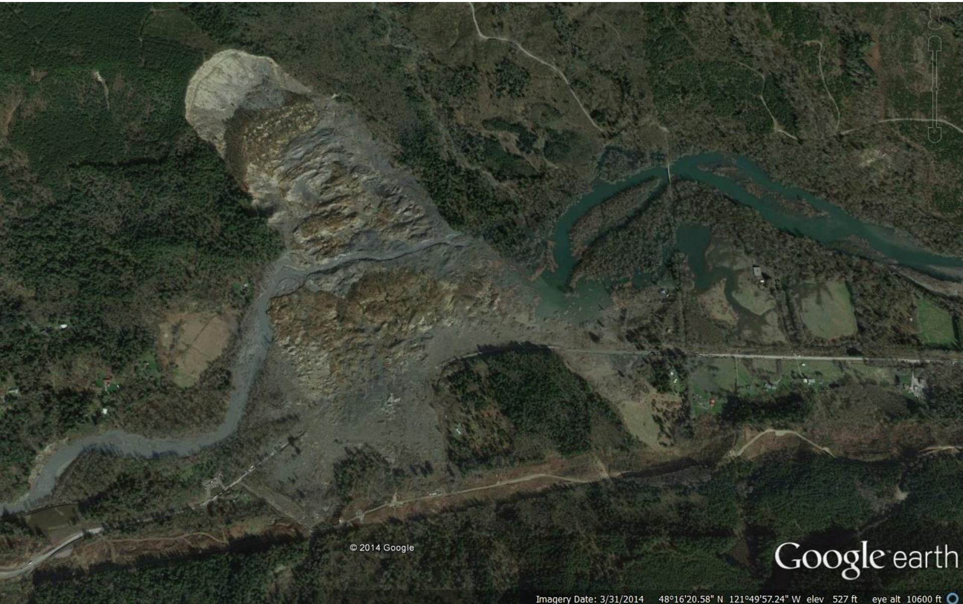
Google Earth Image (March 31, 2014) – approximately 9 days after failure on March 22.
