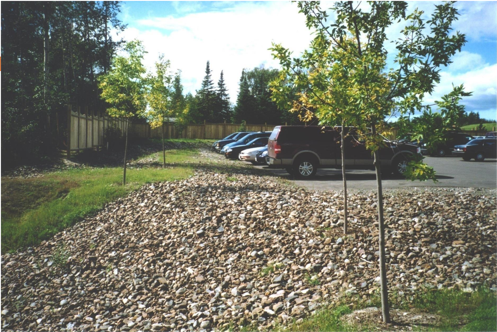
Channel (LHS) and curbless parking lot. TBRH site (Fall 2004).
