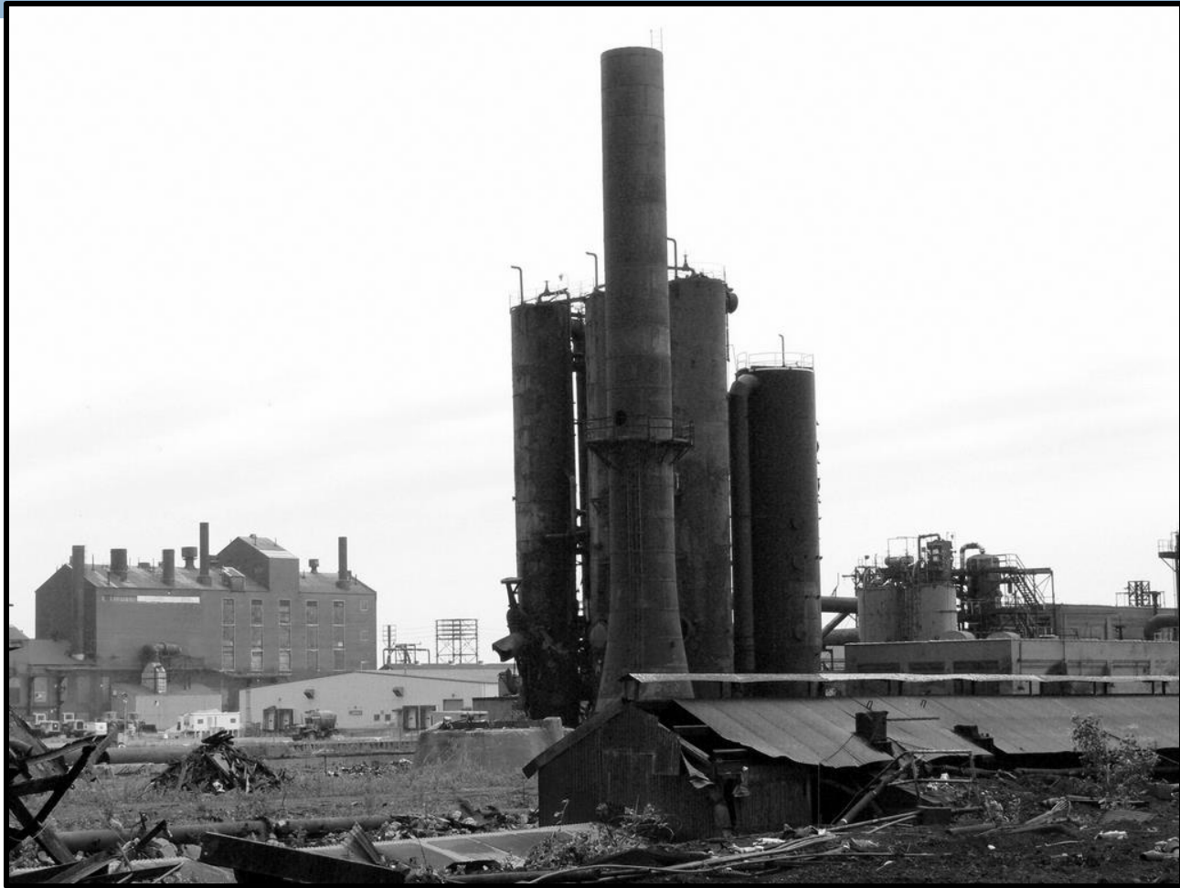
Bethlehem Steel Warehouse
