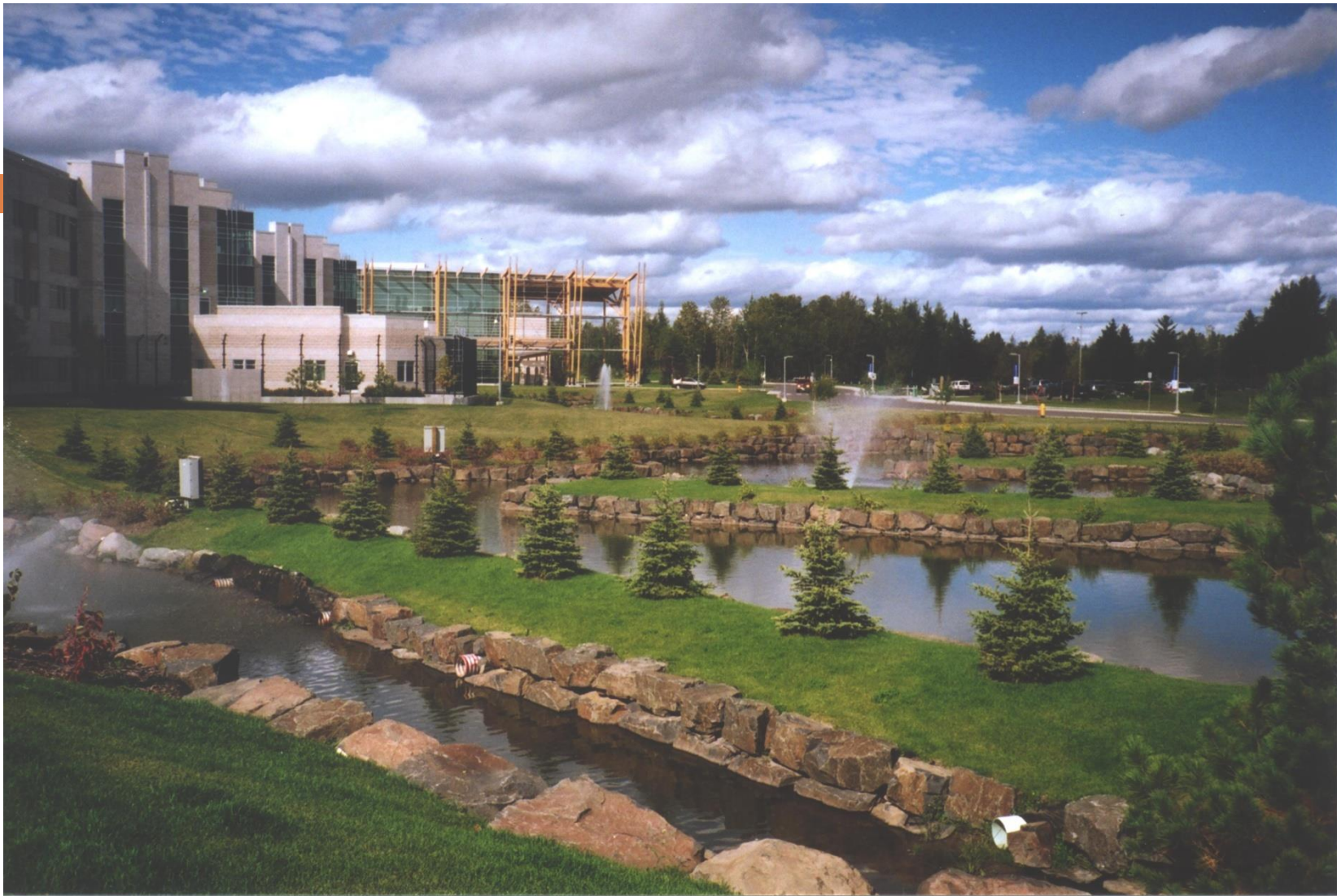
Series of retention ponds along east side of TBRH structure. Fountains to reduce/prevent mosquito larvae. TBRH site (Fall 2004).
