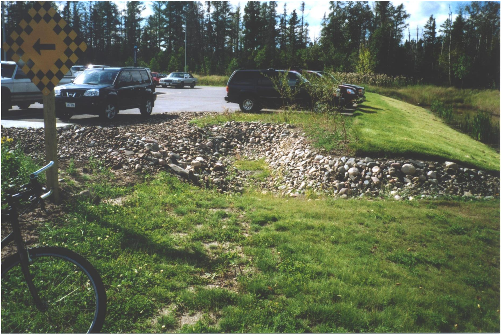
Gravel channel (dry) carries parking lot runoff to holding ponds. TBRH site (Fall 2004).
