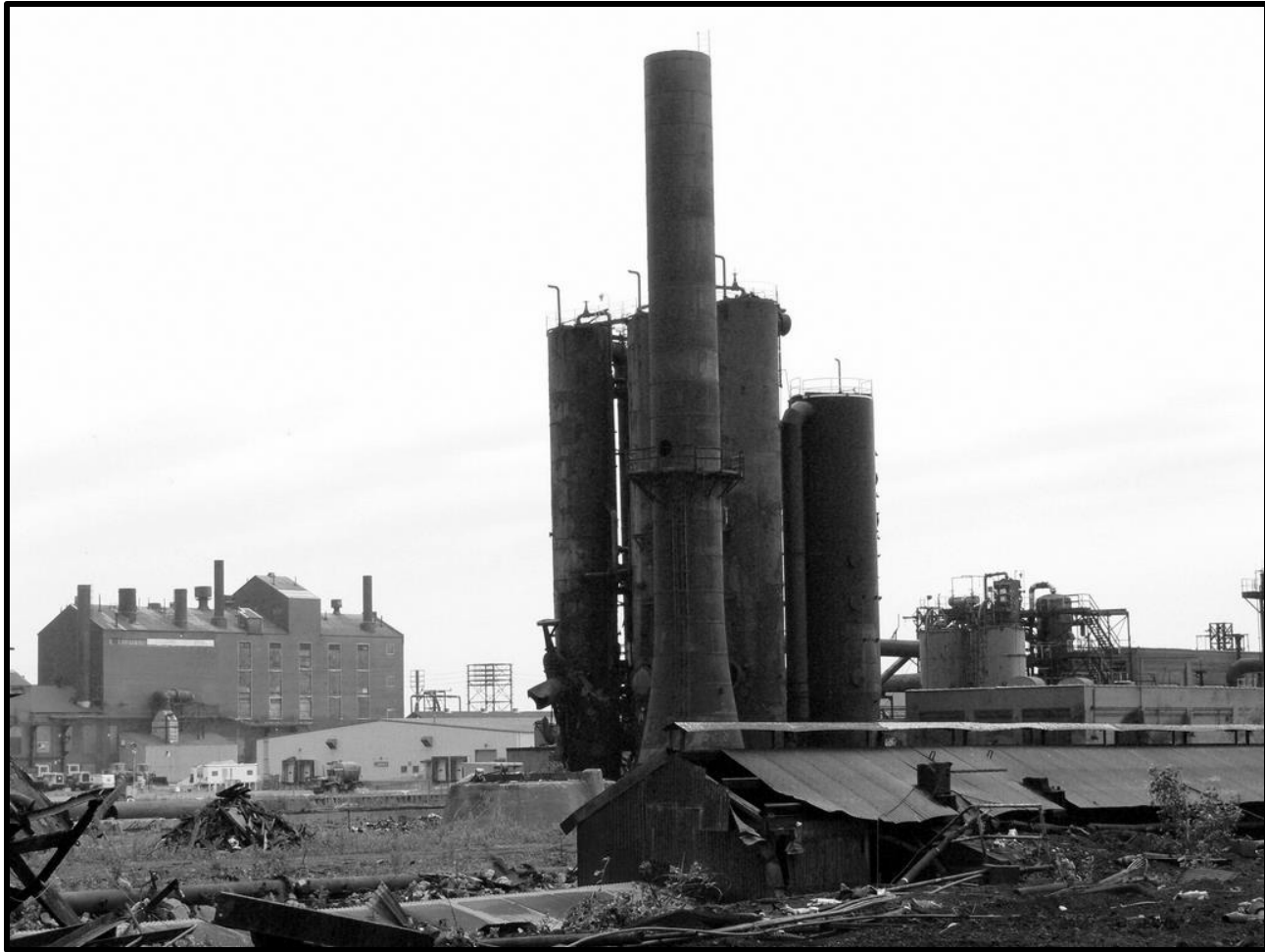
Bethlehem Steel Warehouse
