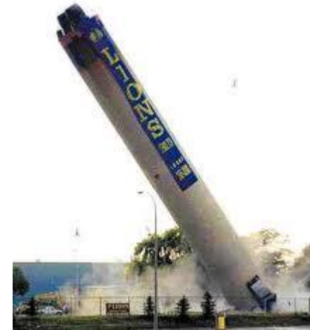
SWARU incinerator (Hamilton), demolished in 2002.
