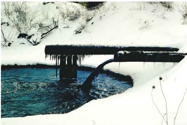
End of pipe (point source) in Great Lakes basin from Dearden and Mitchell (2012)
