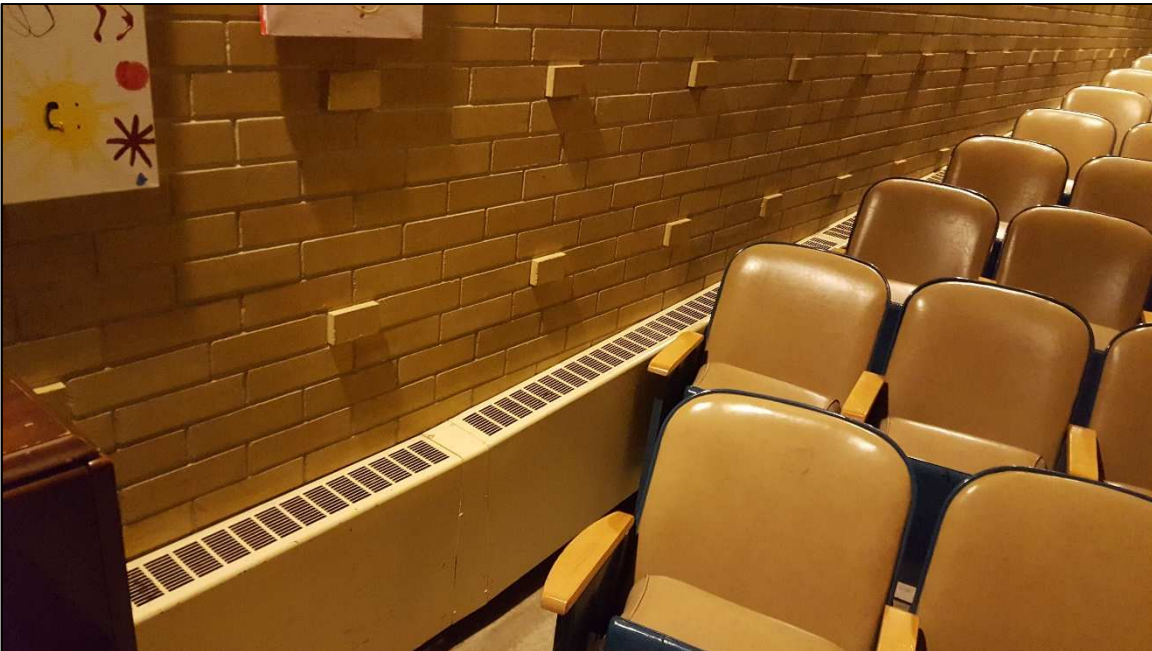
Photo 6 (February 6, 2018) – View of cream paint on heat registers in Auditorium Room 1001 (Sample 202 [Cream]: 4,600 mg/kg lead paint)
