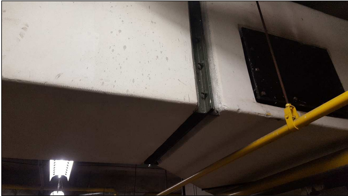
Photo 1 (February 6, 2018) – View of exhaust insulation from the boiler in Boiler Room 0001B (Sample 100A: 50% - 75% Asbestos Containing Material)
