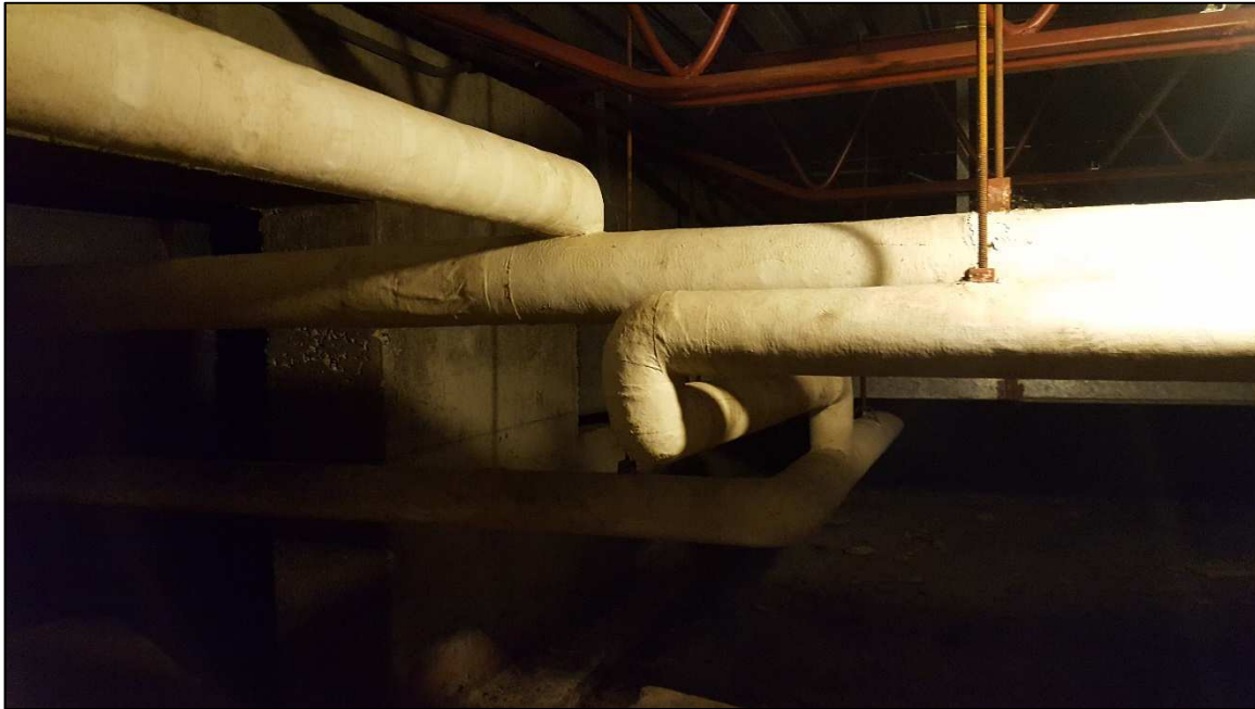
Photo 3 (January 3, 2018) – View of pipe-elbow insulation in crawlspace of east addition (Sample 100E: 50% - 75% Asbestos Containing Material)
