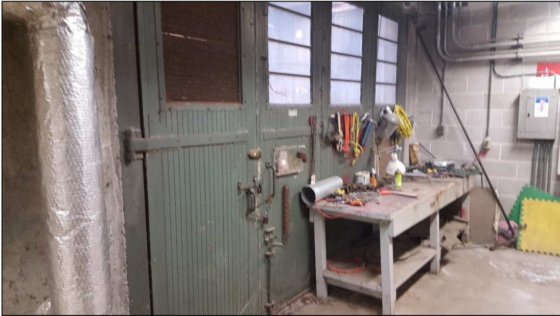
Photo 5 (February 6, 2018) – View of green paint on exterior wooden door in Boiler Room 0001B (Sample 200 (Green): 5,360 mg/kg lead paint)
