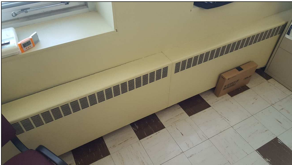
Photo 10 (February 6, 2018) – View of light green wall paint in Room 2029A (Sample 213 [Light Green]: 1,490 mg/kg lead paint)
