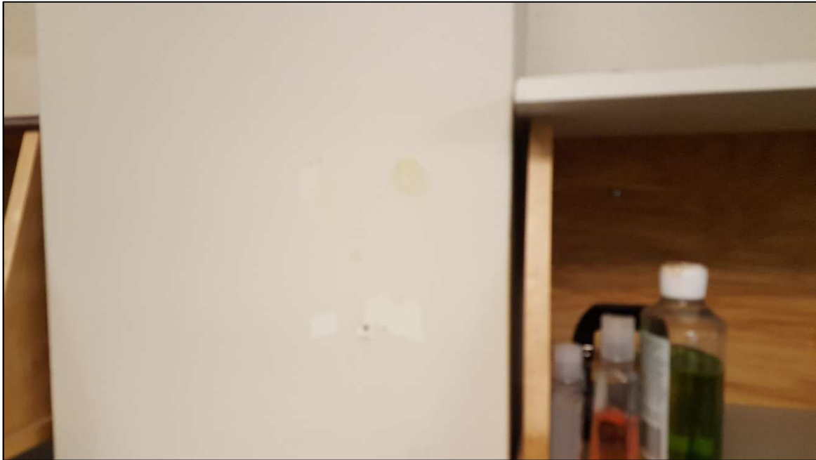
Photo 7 (February 6, 2018) – View white wall paint in Room 1012C (Sample 203 [White]: 2,080 mg/kg lead paint)
