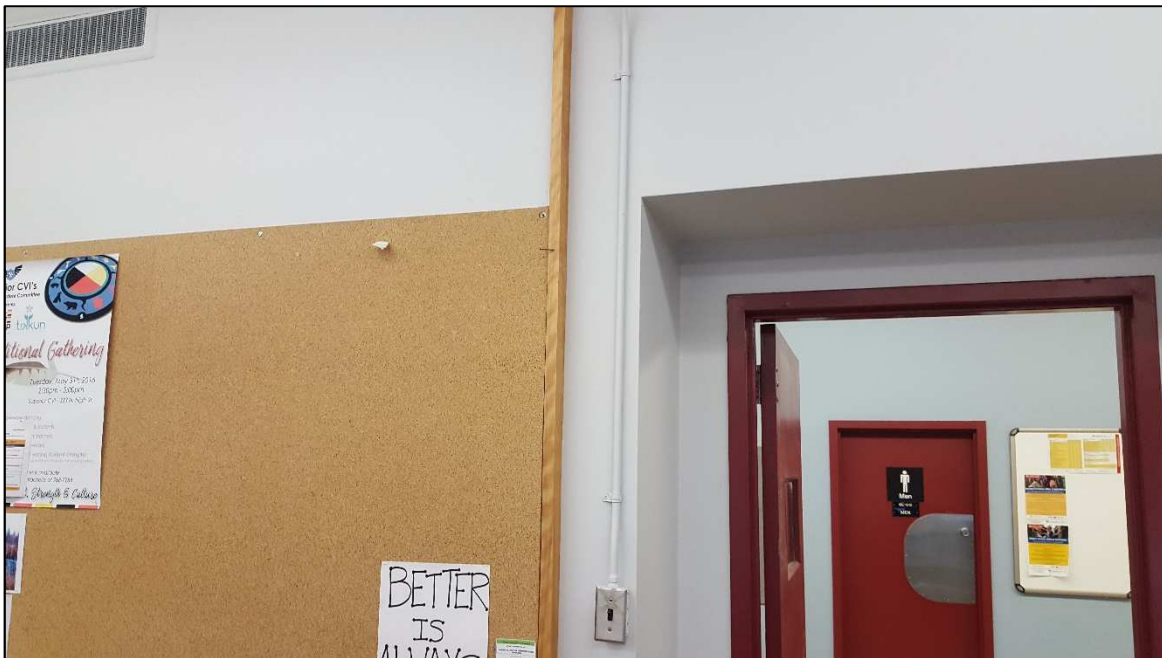
Photo 8 (February 6, 2018) – View of grey paint by door in Room 1022 (Sample 205 [Grey]: 298 mg/kg lead paint)
