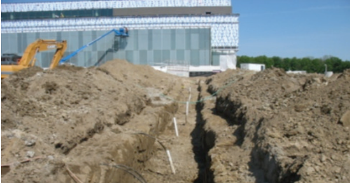
117 boreholes were drilled 330 ft down to create the geothermal system Photo credit: Moriyama & Teshima Architects
